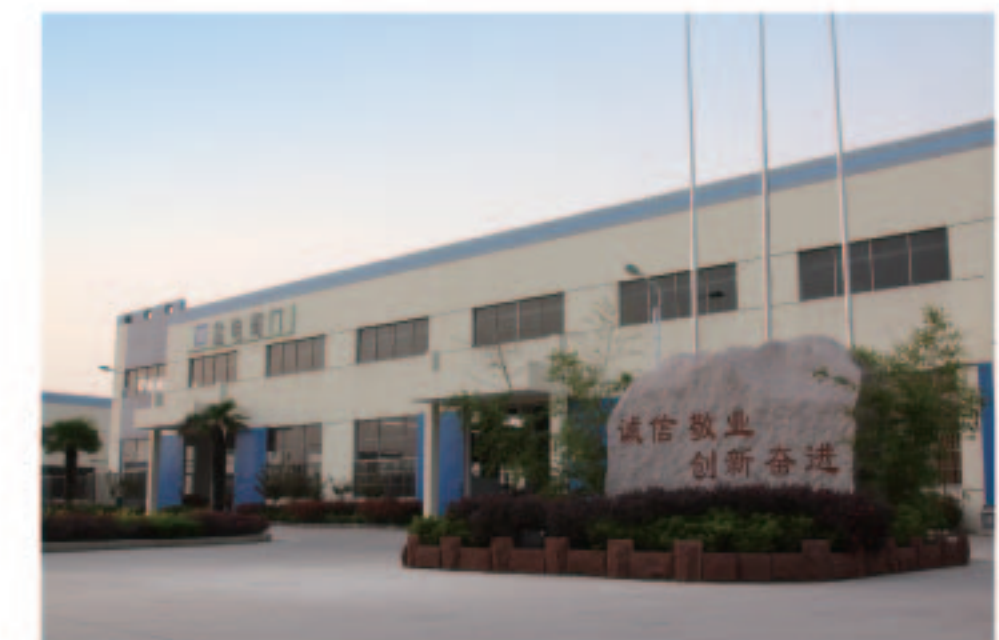
Ball Valve Plant
